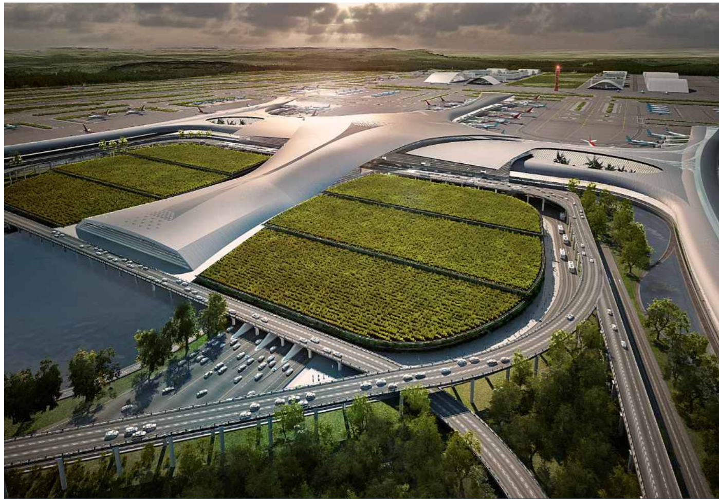
Qingdao New Airport, China
